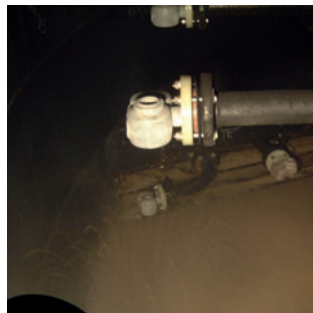
Customized configuration according state-of-art-technologies
