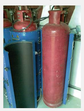
Compressed gas is used during the commissioning and start-up phases of gas turbines, it's critical that a reliable and constant gas supply is available. ISOPAD Hazardous area gas bottle heaters were recently used to guarantee the bottled gas supply met the client's requirements during the start-up ignition sequence at a new plant in Yemen.
